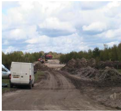
Fig. 2 temporary road diversion
