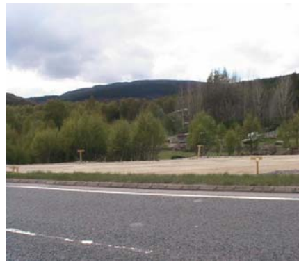
Fig. 3 road diversion viewed from A9
